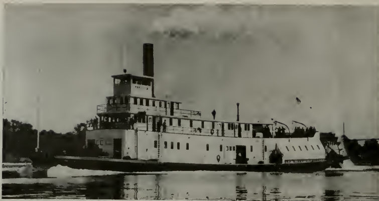
The steamer Portland, built by the Northwest Marine Iron Works, was recently delivered to its owners, the Port of Portland Commission. She will be used for shifting large sea vessels in and about the Portland area waterfront, particularly through the bridges spanning the Willamette River. She will also operate on the Columbia River towing vessels to and from Vancouver, Washington.
